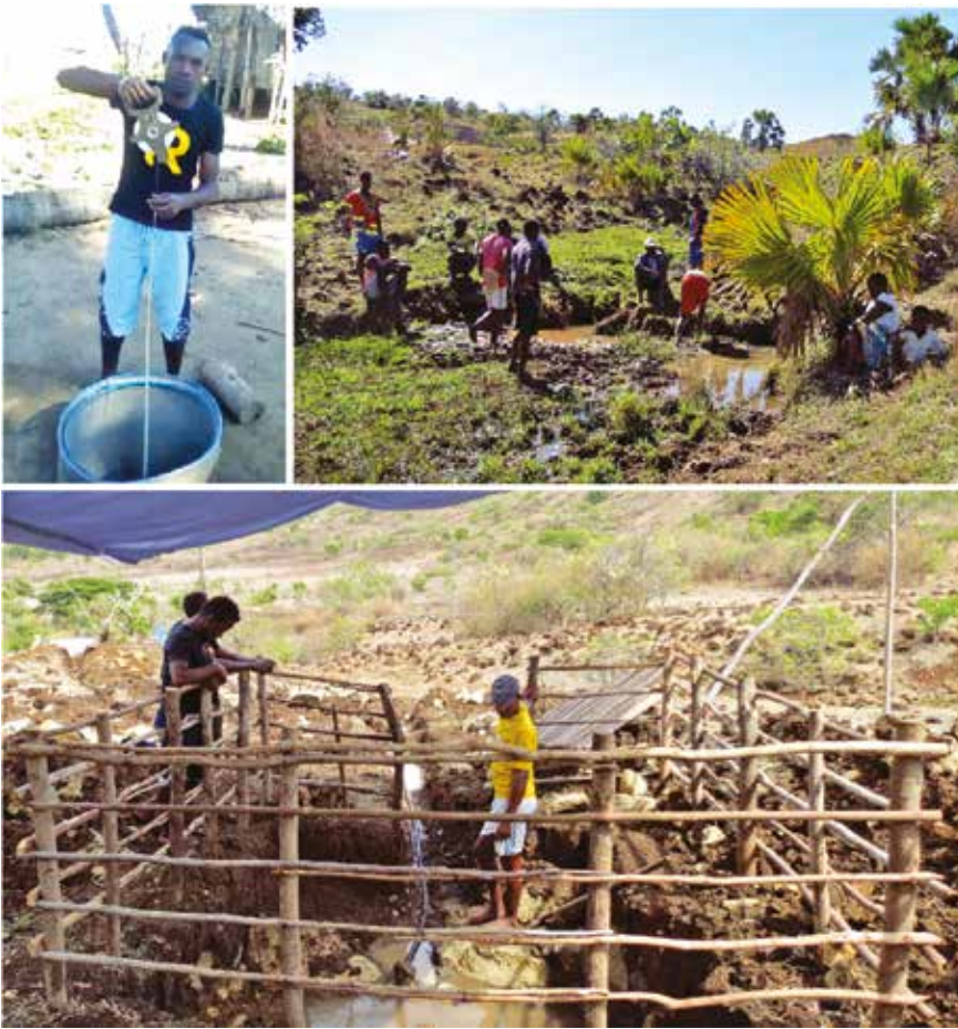
Fig. 4 – Photos taken on Nosy Mitsio island. From top left: a local man measures the well depth; the source WS01 at its natural state; locals engaged in the construction of the water catchment at source WS01.
