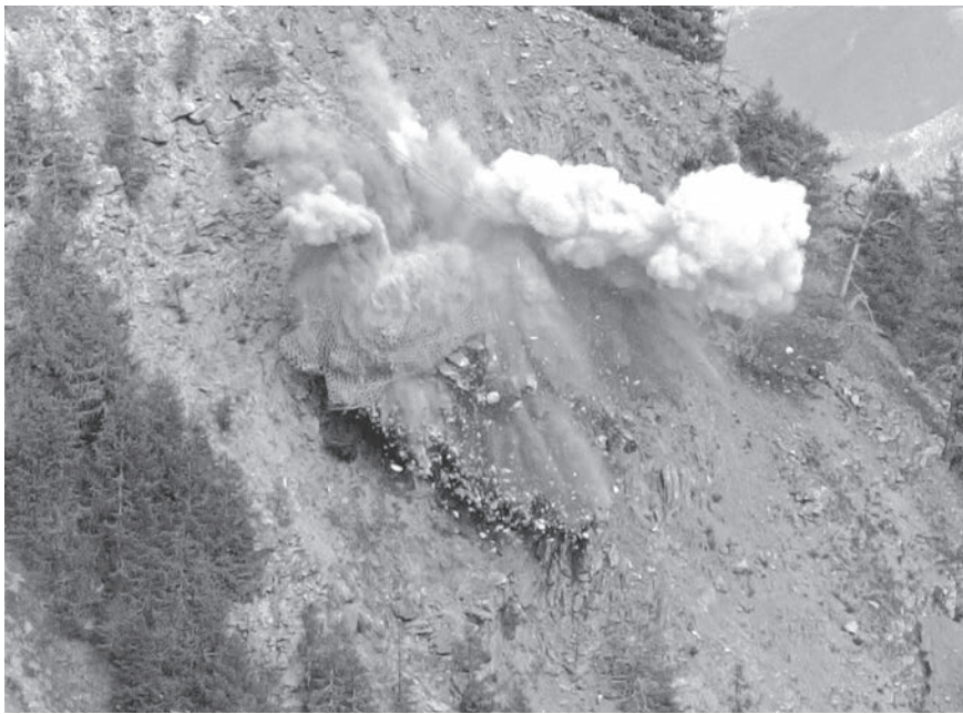
Fig. 4 – Snapshot of the Kastenknott blasting.
