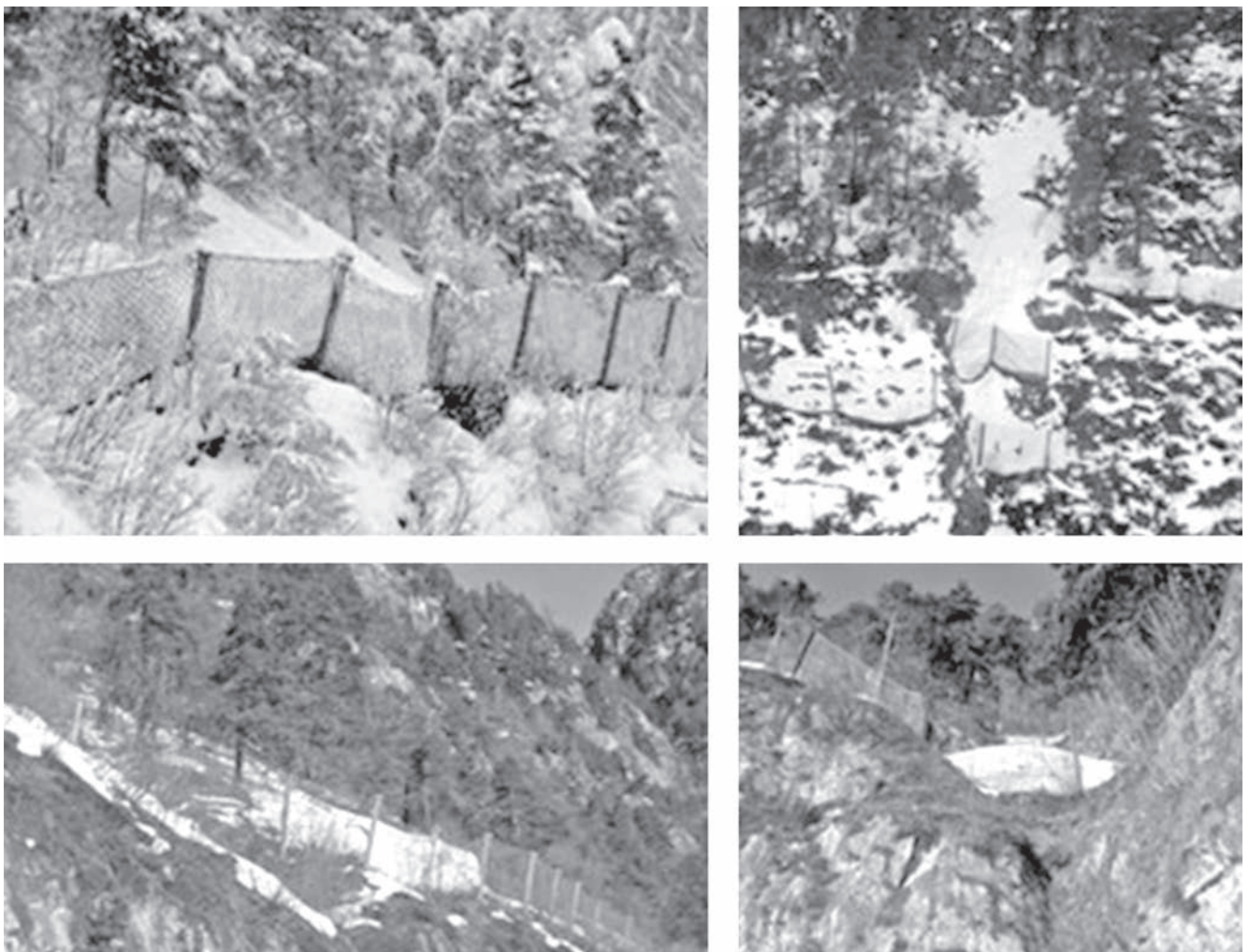
Fig. 3 – Small avalanches of wet snow along the channels obstructing the rockfall barriers; the snow often remains even after the thaw. These phenomena did not occur after the installation of the snow stands.
