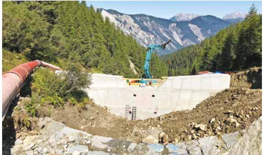
Fig. 12a – Uncovered torrential barrier Leonhardsbach with culverts.
