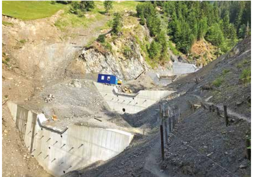
Fig. 8 – Uncovered torrential barrier Toedterbach with outlets.
